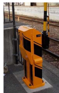
踏切遮断機更新
