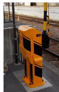
踏切遮断機更新
