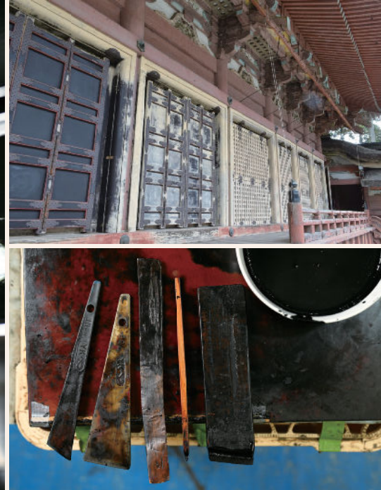
TOP: Damaged fitting prior to restoration BOTTOM: Tools for lacquering
