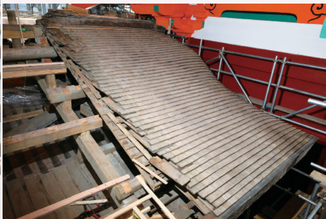
The shingles believed to be from the Edo period that remain on the north and south sides of the cloister
