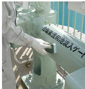
Example of onsite application of photocatalytic cover coating to equipment
