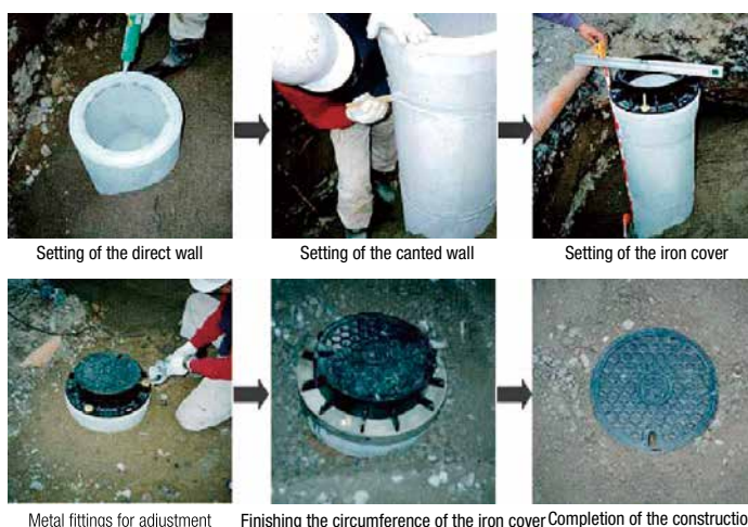
Metal fittings for adjustment Finishing the circumference of the iron cover Completion of the construction
