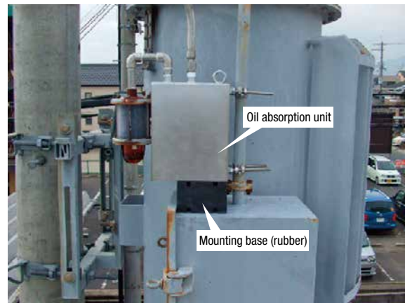
Installation example No. 2 of Spouting Oil Adsorption Unit for Electrical Equipment Filled with Oil
