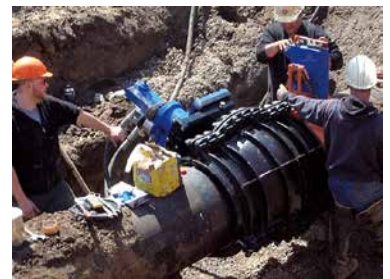
Valve installation with S-GATE (end mill under a pressure installation system)
