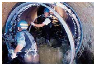
Construction site where the SPR method is implemented
