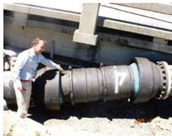
SUPER FLEX incurred no damage during the Loma Prieta Earthquake.
