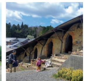
One local potter's facilities in the Shigaraki pottery district (left) and an old decommissioned climbing kiln (right) which used the natural slope to distribute heat to upper chambers.
