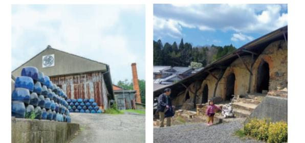
One local potter's facilities in the Shigaraki pottery district (left) and an old decommissioned climbing kiln (right) which used the natural slope to distribute heat to upper chambers.
