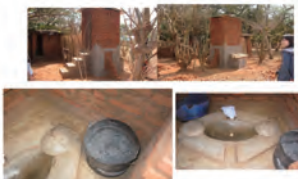
Fig. T5-1 A urine feces diversion toilet for hygiene
