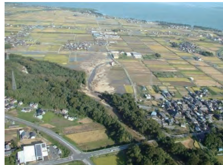
Fig. 4-11-3 Takashima City after the Typhoon No. 18 in 2013 Collapses at the Kamo River
