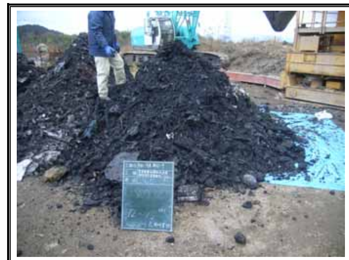
掘削廃棄物土(GL-12.00~15.00m)
