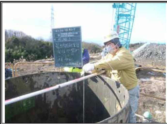
掘削深度確認 (GL-24.00m)
