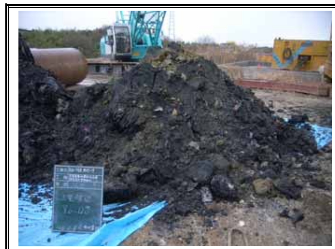
掘削廃棄物土(GL-9.00 ~ -12.30m)
