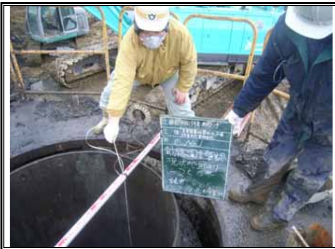
掘削深度確認 (GL-25.00m)
