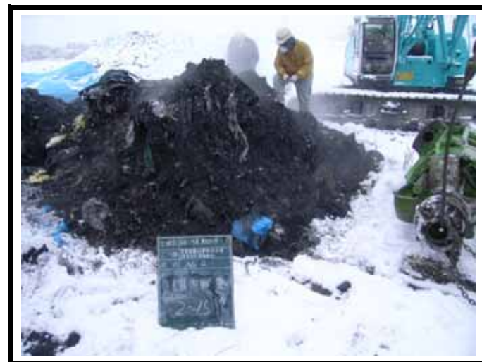
掘削廃棄物土(GL-12.00~15.00m)
