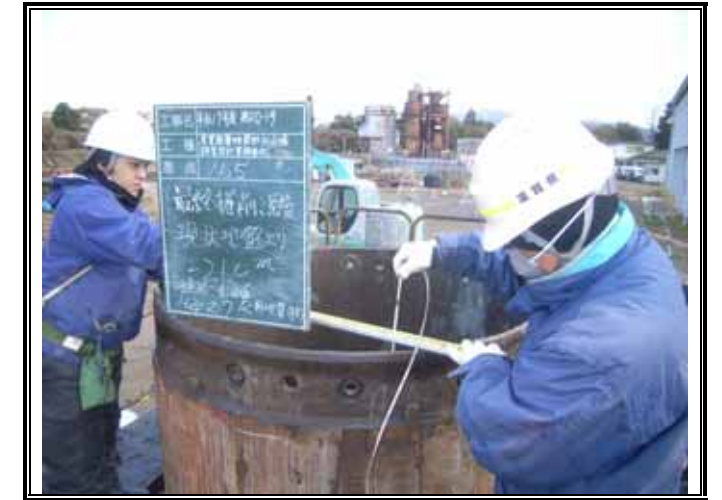
掘削深度確認 (GL-21.00m)
