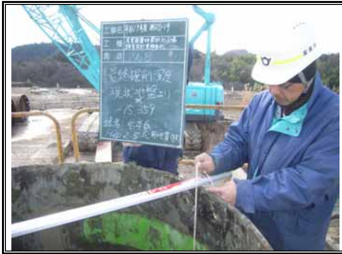
掘削深度確認 (GL-15.35m)
