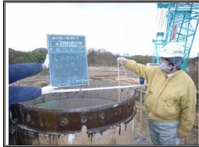
掘削深度確認(GL-17.80m)
