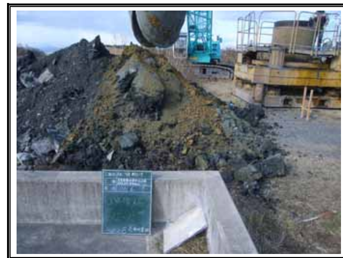
掘削廃棄物土(GL-12.00~15.00m)
