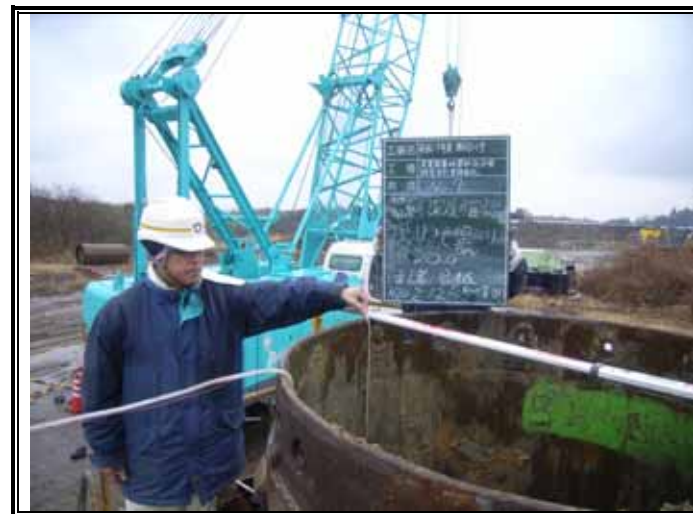
掘削深度確認(GL-20.00m)
