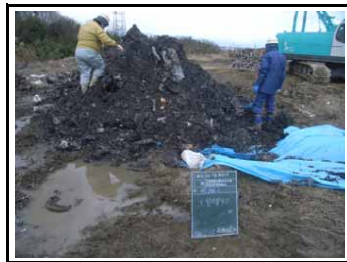
掘削廃棄物土(GL-12.00~15.00m)
