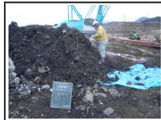
掘削廃棄物土(GL-12.00~15.00m)
