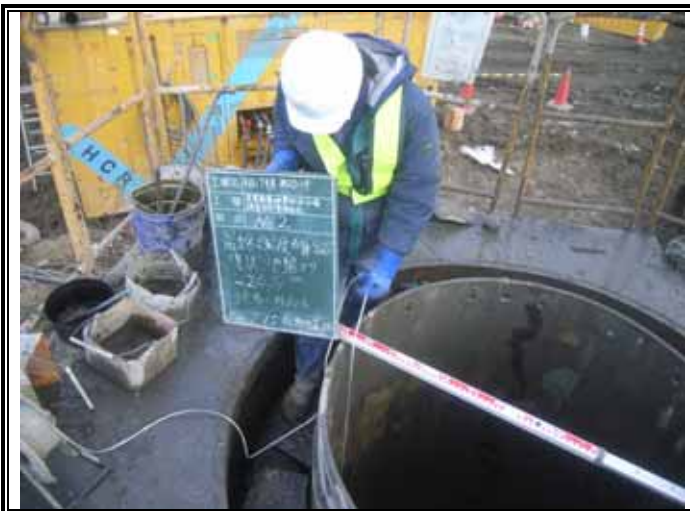
掘削深度確認 (GL-24.80m)
