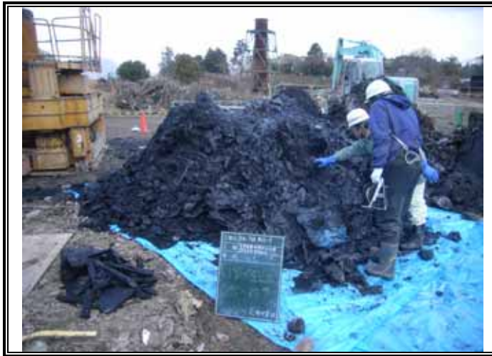
掘削廃棄物土 (GL-15.00 ~ 18.00m)
