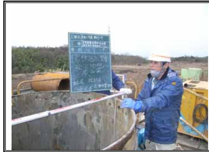
掘削深度確認(GL-14.20m)
