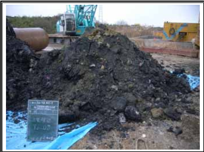
掘削廃棄物土 (GL-9.00 ~ -12.30m)
