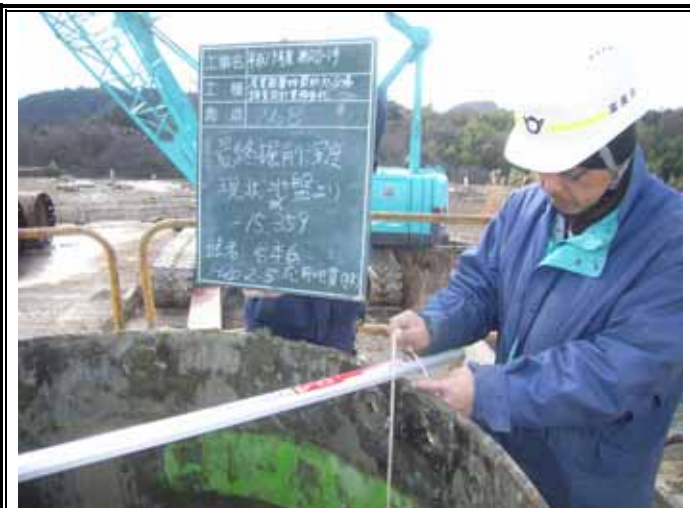
掘削深度確認 (GL-15.35m)
